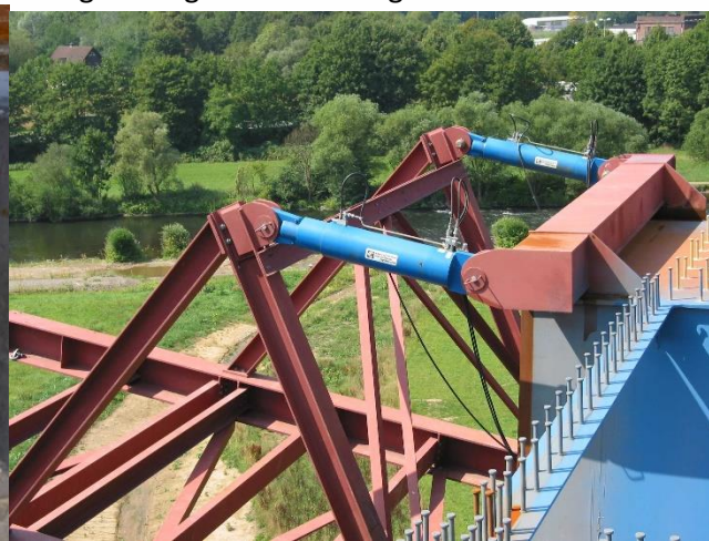
Launching-nose lifting unit Hydraulic lifting unit bolted nose
