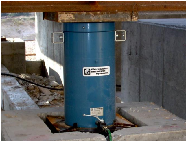
Hydraulic jack With adjustable locking ring
